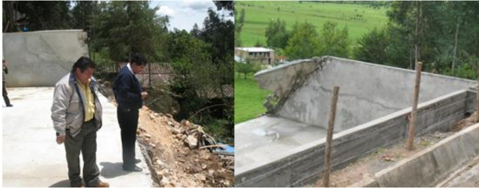
Figura 7. Colapso del reservorio Huayrapongo (Mosqueira, 2014)
