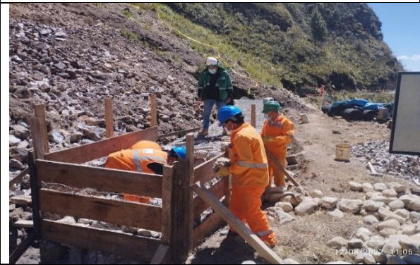
24 SUMINISTRO E INST. GAVION CAJA (2.0x1.0x1.0m), MALLA 10x12, DIAM. 2.7mm, 3 ZN+PVC
