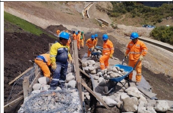
24 SUMINISTRO E INST. GAVION CAJA (2.0x1.0x1.0m), MALLA 10x12, DIAM. 2.7mm, 3 ZN+PVC
